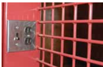
Built-in electric system
