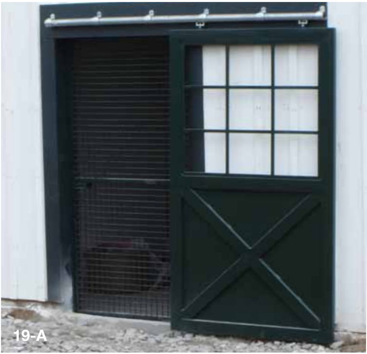
Sliding exterior door with pre-hung crosshatch mesh rear screen. Window on top and crossbuck design on bottom.
