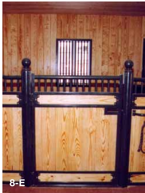
8-E Steel-framed hinged door with low front and wood bottom, decorative center rail and bedding guard. Painted steel ball finials.
