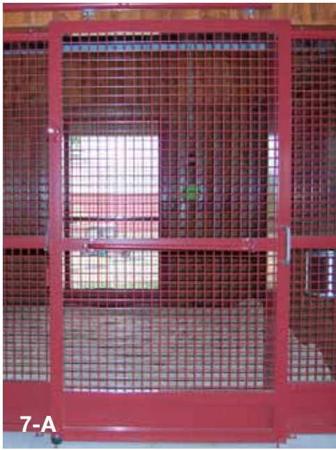
7-A Steel-framed sliding door with crosshatch mesh top and bottom. 12-inch bedding guard.
