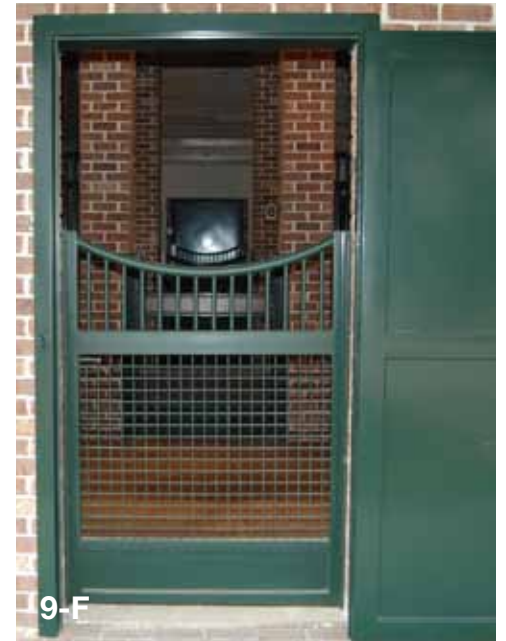
Steel-framed half-screen with yoke cutout, steel bars, crosshatch mesh, latching mechanism, and bedding guard.
