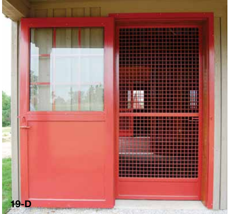
Exterior hinged door with pre-hung crosshatch mesh rear screen and bedding guard. Glass window on top; steel bottom.
