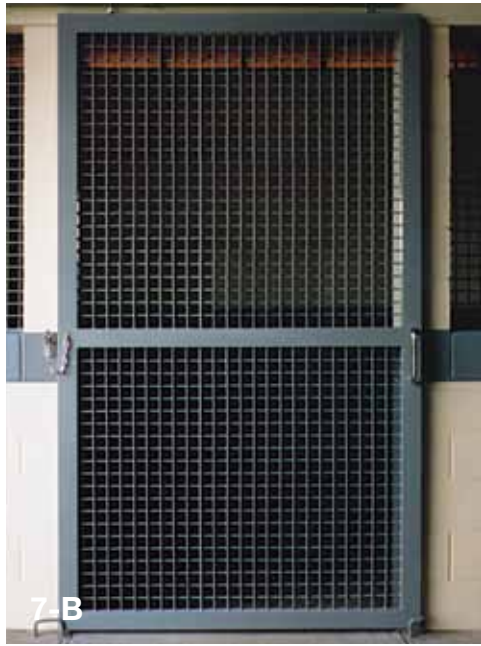
7-B Steel-framed sliding door with crosshatch mesh top and bottom. No bedding guard.
