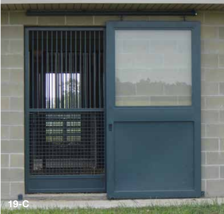
Sliding exterior door with pre-hung rear screen (bar grills over crosshatch mesh with bedding guard). Glass window on top; steel bottom.
